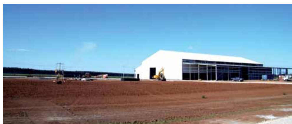
Below: Construction on the new cotton gin is well under way.
